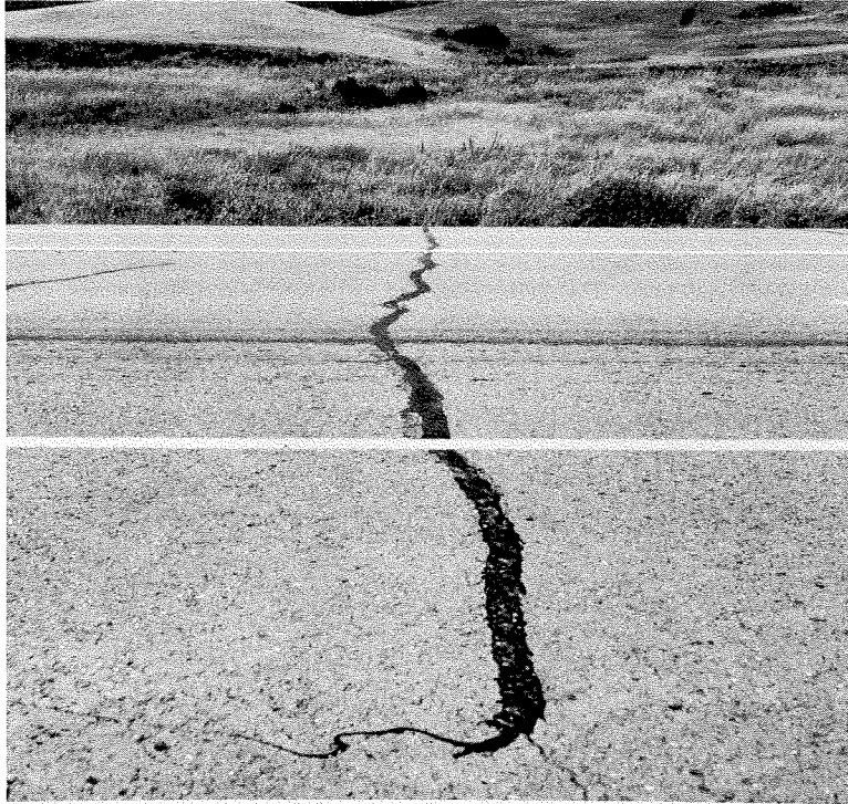
Figure 15 — Location near Peace River, Alberta. Transverse cracks extend through paved shoulders when main pavement and paved shoulders contain 150/200 or 200/300 penetration asphalt.
