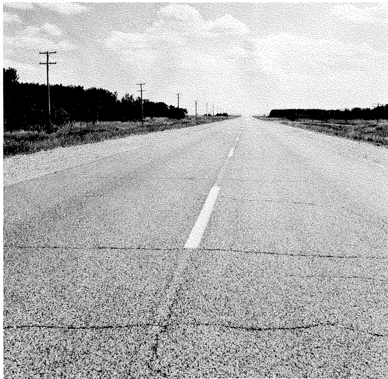
Figure 22 — 150/200 Penetration Pavement, located near Brandon, Manitoba, constructed in 1963.
