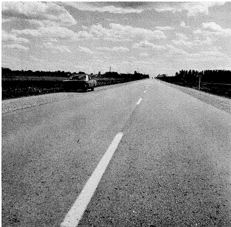
Figure 24 — 300/400 Penetration (SC 6) Pavement, located near Neepawa, Manitoba, constructed in 1965.
