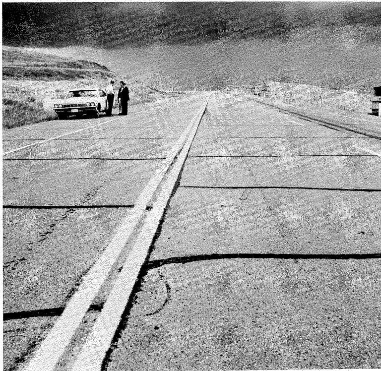
Figure 14 — 150/200 Penetration Pavement, located near Peace River, Alberta, constructed in 1963.
