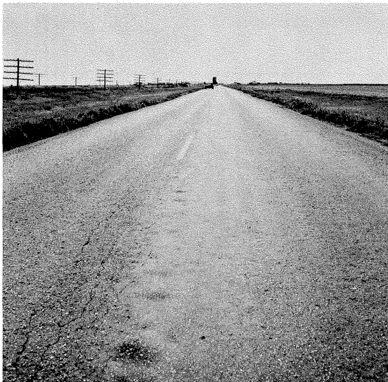
Figure 20 — Complete absence of periodic well-marked transverse cracks in SC 2 road mix \frac{3}{4} -inch thick laid directly on subgrade, located near Regina, Saskatchewan.
