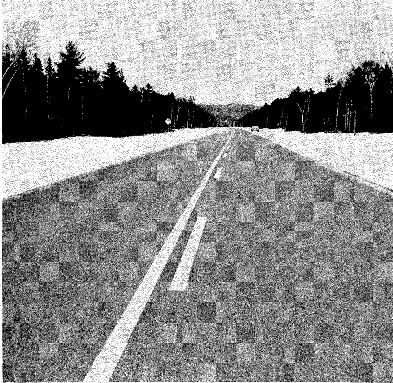
Figure 9 — 150/200 Penetration Pavement, located about 40 miles north of Sault Ste. Marie, Ontario, constructed in 1963.
