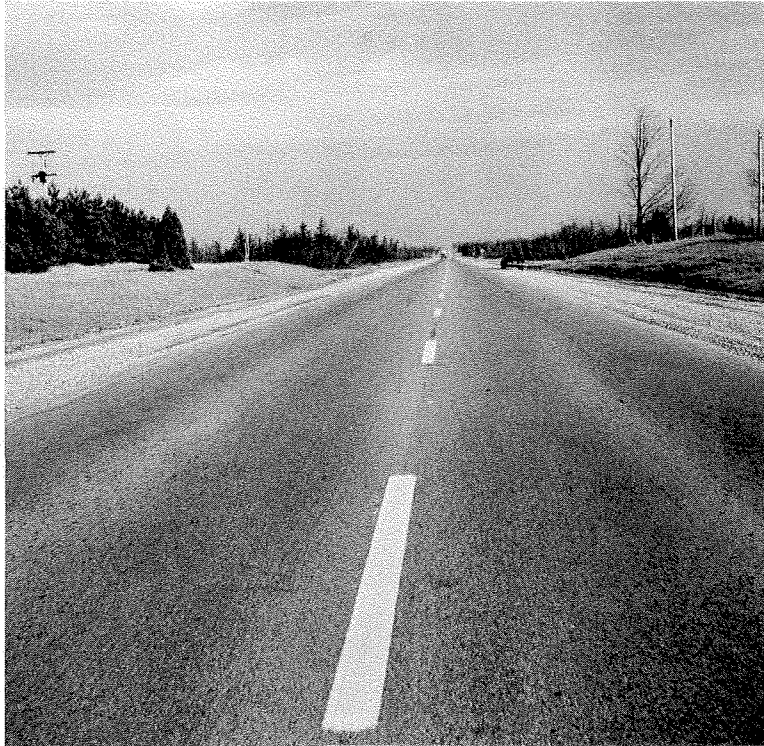
Figure 11 — 150/200 Penetration Pavement, located west of Orangeville, Ontario. Four years old.
