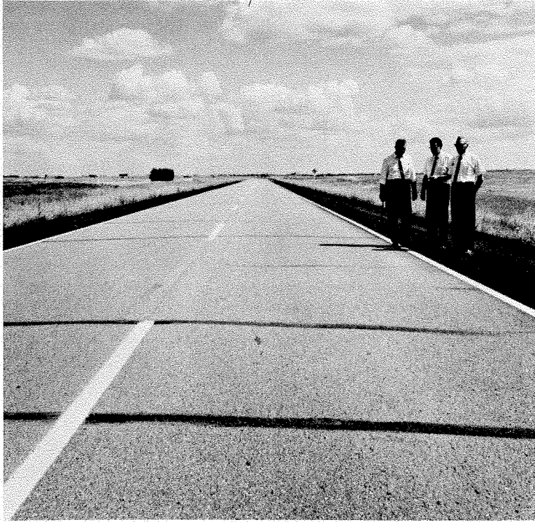
Figure 17 — 150/200 Penetration Pavement, located near Saskatoon, Saskatchewan, constructed in 1959.
