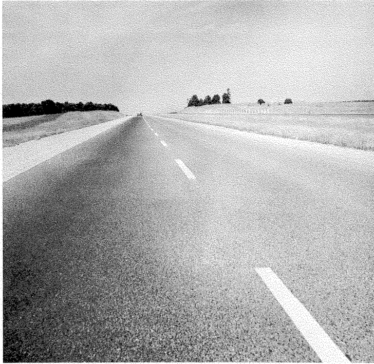
Figure 13 — 85/100 Penetration Pavement, located west of Galt, Ontario. Four years old.
