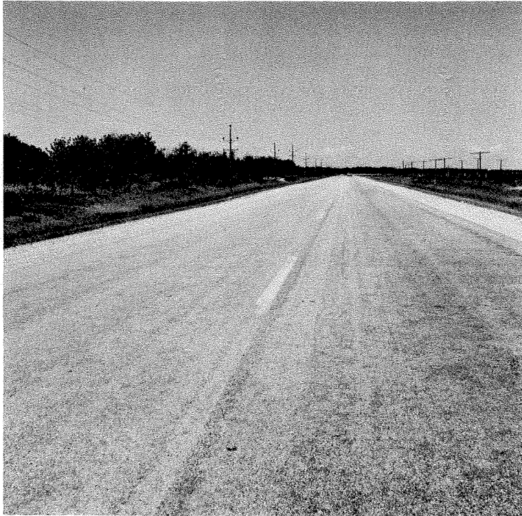
Figure 23 — 300/400 Penetration (SC 6) Pavement, located near Portage la Prairie, Manitoba, constructed in 1952.
