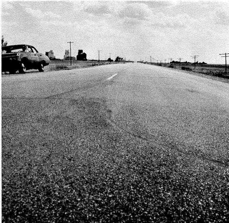
Figure 18 — Bump has developed at each transverse crack in hot-mix pavement near Regina, Saskatchewan.
