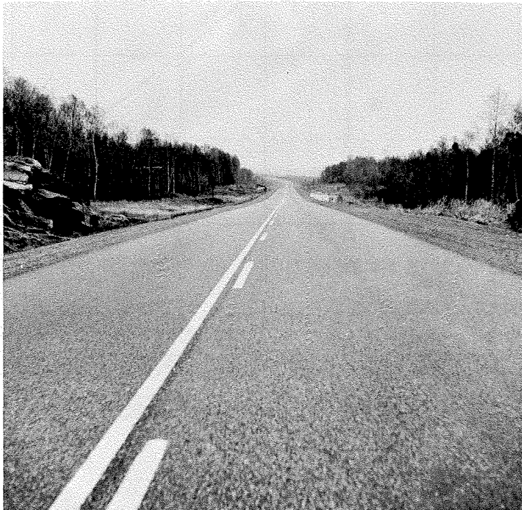
Figure 6 — 150/200 Penetration Pavement, located about 110 miles east of Port Arthur, Ontario, constructed in 1960.
