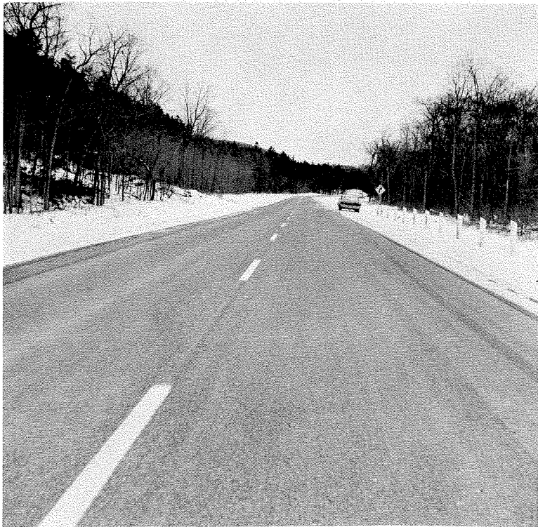
Figure 8 — 150/200 Penetration Pavement, located about 30 miles north of Sault Ste. Marie, Ontario, constructed in 1962.
