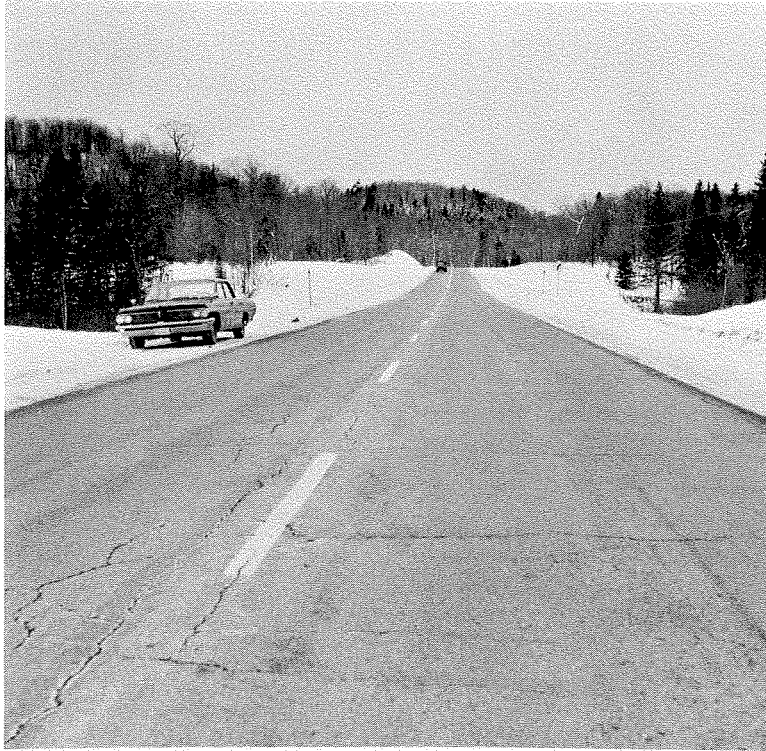
Figure 7 — 85/100 Penetration Pavement, located about 20 miles north of Sault Ste. Marie, Ontario, constructed in 1960.
