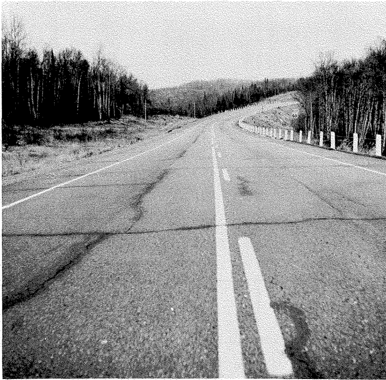
Figure 5 — 85/100 Penetration Pavement, located about 120 miles east of Port Arthur, Ontario, constructed in 1961.
