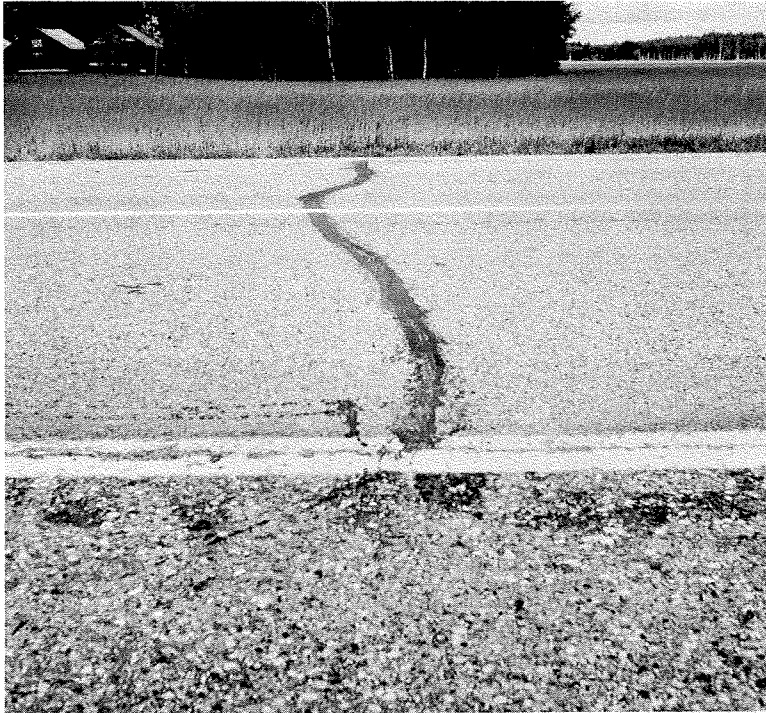
Figure 16 — Location near Peace River, Alberta. Transverse cracks in 150/200 or 200/300 penetration main pavement do not extend into the paved shoulder constructed with MC 2 or MC 3 liquid asphalt.
