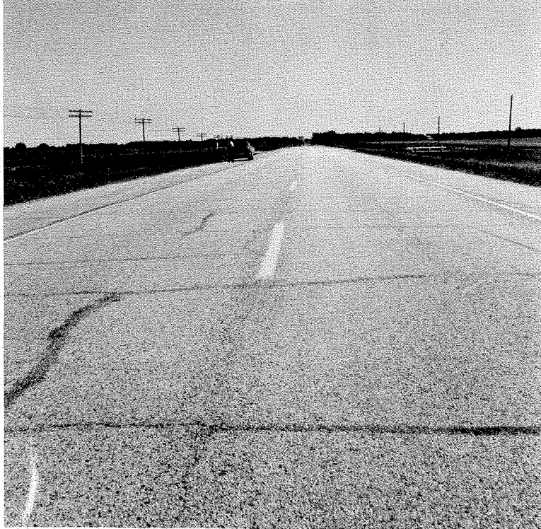
Figure 21 — 150/200 Penetration Pavement, located near Portage La Prairie, Manitoba, constructed in 1960.
