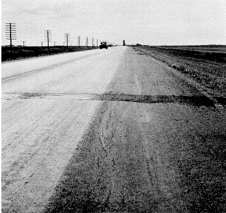
Figure 19 — Well-defined transverse cracks from 100 to 150 feet apart in pavement consisting of 16 inches of granular base and a surface treatment, located near Regina, Saskatchewan.
