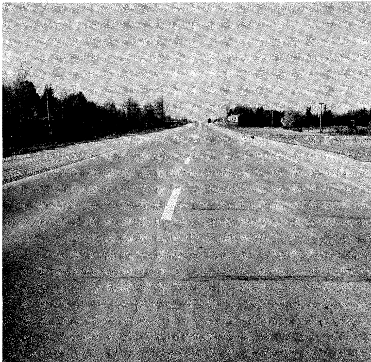
Figure 12 — 85/100 Penetration Pavement in right lane, 150/200 Penetration Pavement in left lane, located west of Orangeville Ontario. Four years old.
