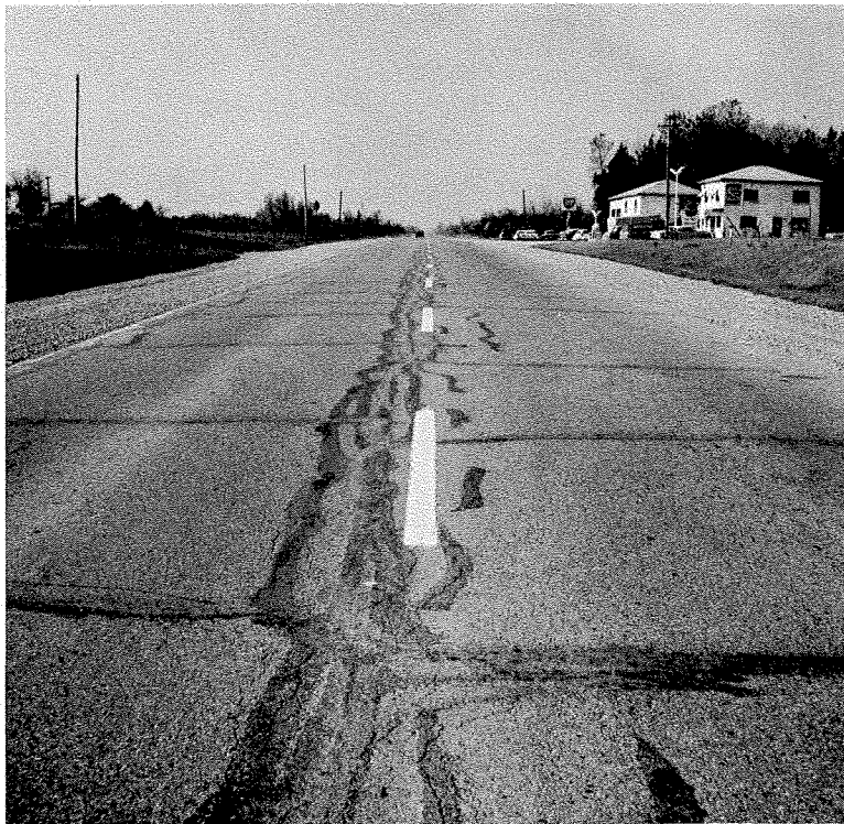
Figure 10 — 85/100 Penetration Pavement, located west of Orangeville, Ontario, Four years old.
